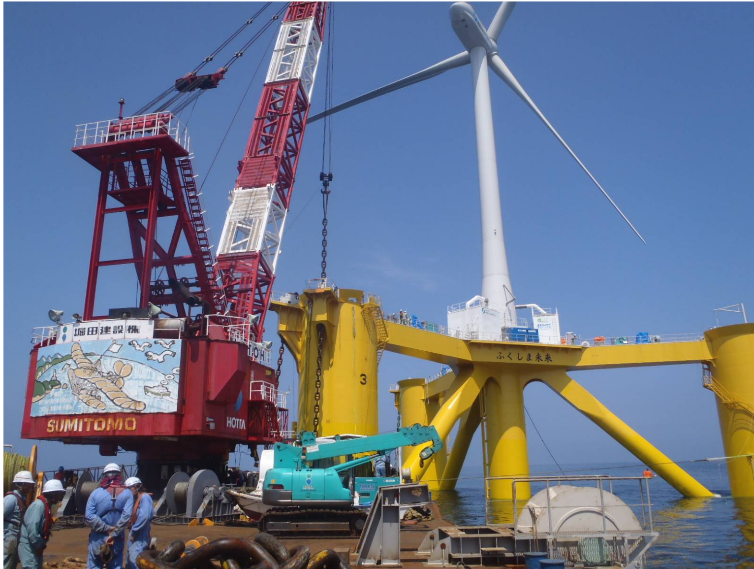
Connecting chain to the floater (Photo credit: SSE JV)
