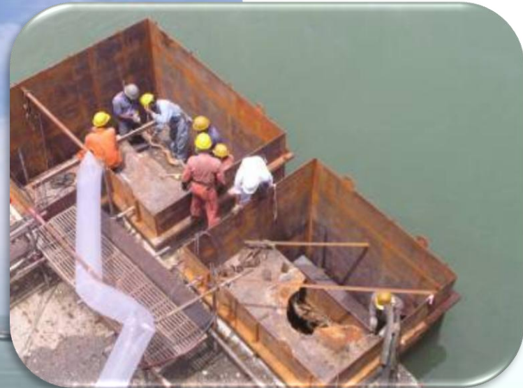
DAMAGE REPAIRS TO HER SUBMERGED MAT ATTENDED WHILE AFLOAT
