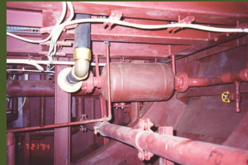
Fuel Oil Pump Isolation & Acoustic Filter
